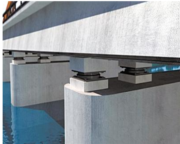
An illustration showing bridge bearings are in place under the bridge deck beam and above the pillars
