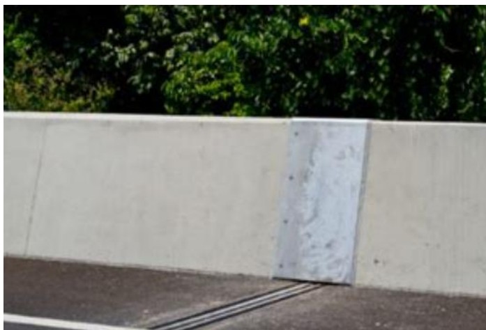
Cover plate over the modular expansion joint in the parapet area
