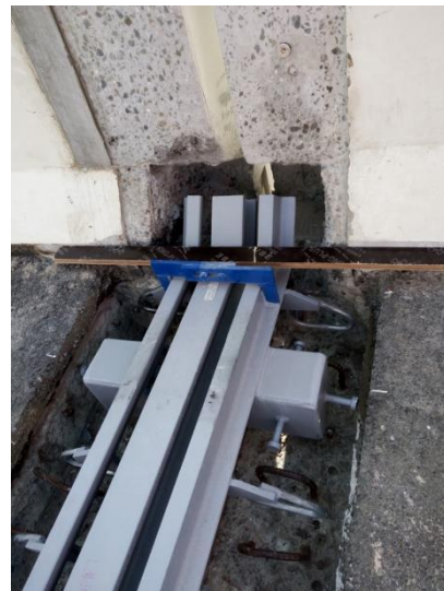
how the uturn extends into the reserved void in the parapet
