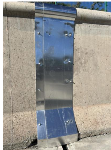
Cover plate over the modular expansion joint in the parapet area
