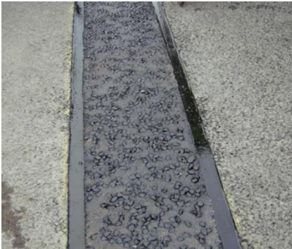
Asphaltic Plug expansion Joint
