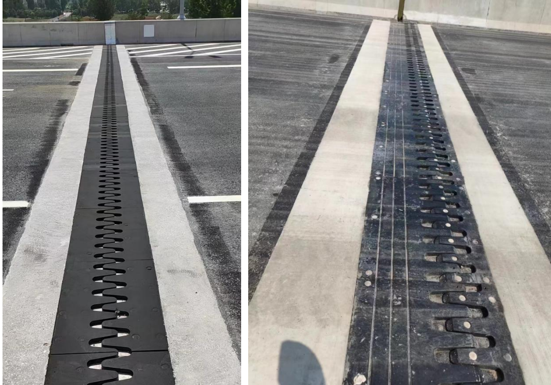
A simple set of images comparing the difference between a cantilever finger joint (left) and a supported finger joint (right)
