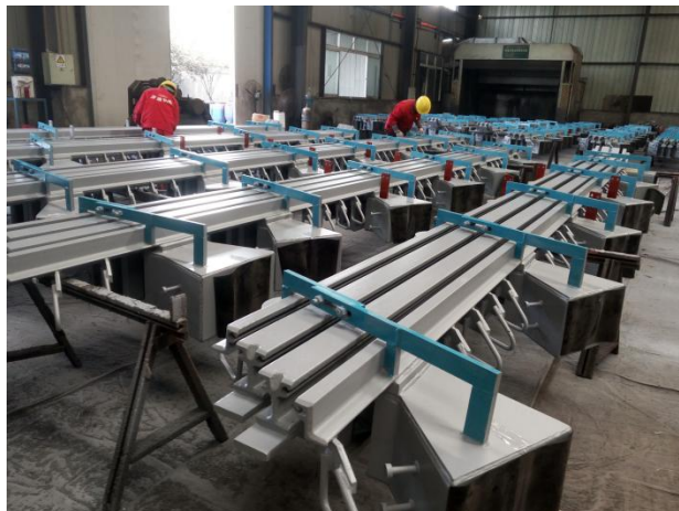
Painting of modular expansion joint at IEC workshop for NOH2 project in Doha Qatar, 2018
