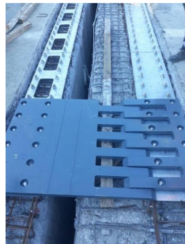
Numerous such finger joints have been supplied and installed by IEC in China (mostly supported structure)
