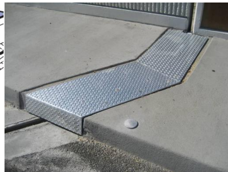
A typical design of a cover plate for the sidewalk area over the expansion joint upturn
