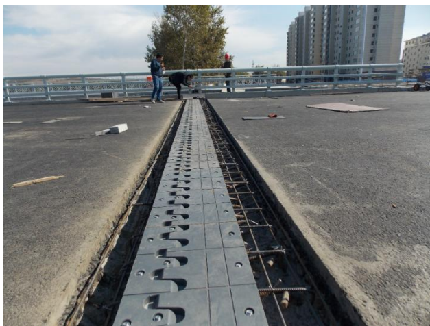
Numerous such finger joints have been supplied and installed by IEC in China (mostly supported structure)
