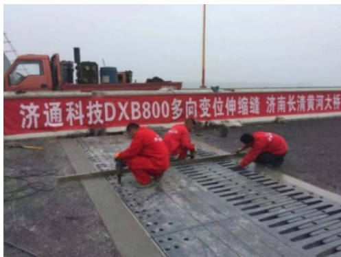
IEC supplied a 800mm movement DXB finger joint system for Brive over Huanghe River in Jiqing, Shandong, China
