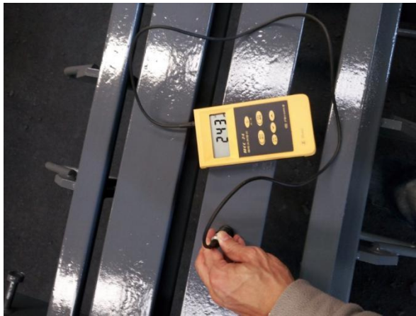
paint film thickness 243 microns (C5-MI) for E-ring road project in Doha Qatar, 2018
