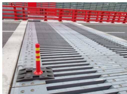
IEC supplied a 800mm movement DXB finger joint system for Brive over Huanghe River in Jiqing, Shandong, China
