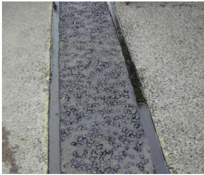
Asphaltic Plug expansion Joint
