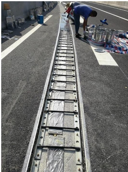
Installation of PUF joint for Changshen Expressway, Hangzhou Section in Zhejiang, China 2022
