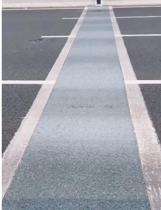
Installation of PUF joint for Changshen Expressway, Hangzhou Section in Zhejiang, China 2022
