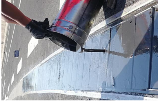
PUF polyurethane joint supplied and installed by IEC at Yuguang expressway, Chongqing, China 2020
