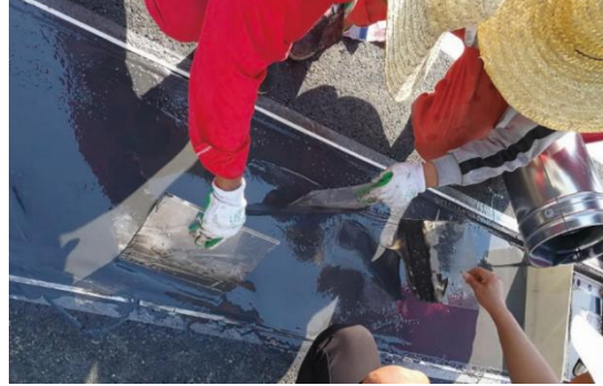
PUF polyurethane joint supplied and installed by IEC at Yuguang expressway, Chongqing, China 2020
