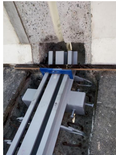
how the upturn extends into the reserved void in the parapet
