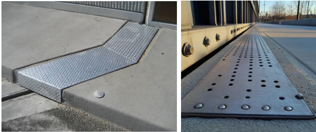
A typical design of a cover plate for the sidewalk area over the expansion joint upturn
