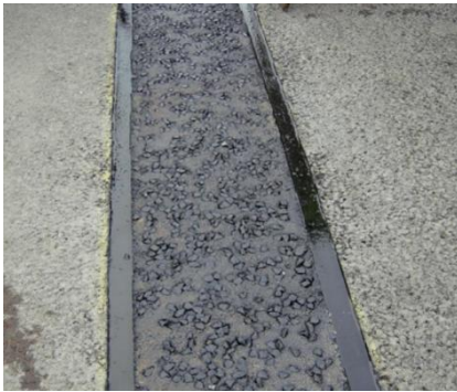
Flexible Plug Expansion Joint
