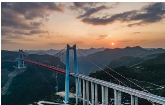
Qingshui River Bridge, Guizhou Province, China (1600mm movement)
