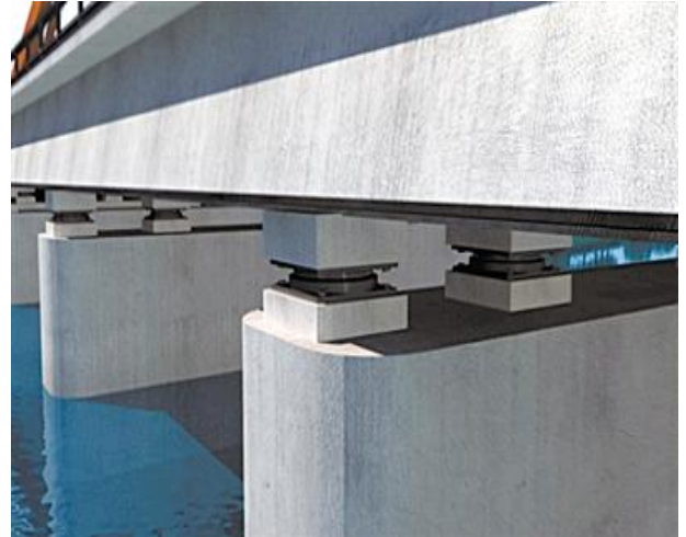
Role of bridge bearings (right on piers)
